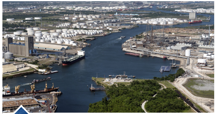
Onshore petroleum facilities along the Houston ship channel.
