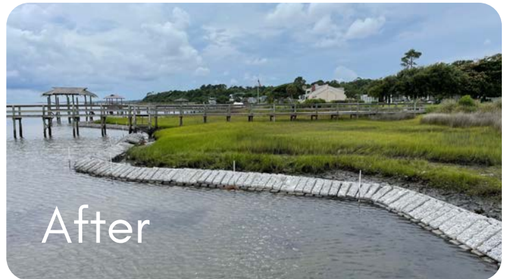
QuickReef™ units from Native Shorelines, a division of Restoration Systems, LLC, are made up of a mixture of oyster shells and limestone marl to protect shorelines from erosion and provide valuable oyster and fish habitat.
