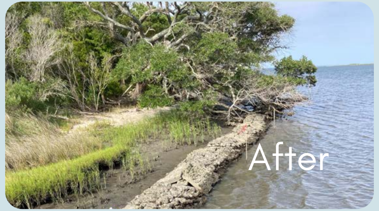
Bogue Sound shoreline with an offshore sill built with bags of recycled oyster shells and Native Shorelines, a division of Restoration Systems, LLC, QuickReef™ structures.
