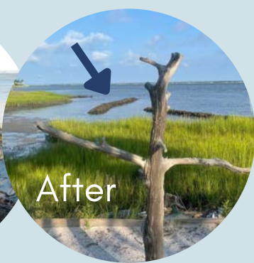
Living Shoreline with offshore oyster reefs, built in 2014, and planted with saltmarsh grasses at Trinity Center in Pine Knoll Shores.
