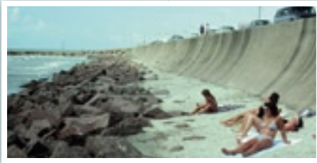
Galveston, TX seawall, Hurricane Rita 2005. Photo courtesy U.S. Army Corps of Engineers.
