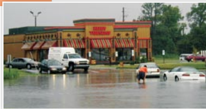
The state's coastal stormwater program has failed to protect the public's safety as this photo of a shopping center after a moderate rain shows. Numerous detention ponds permitted under the program failed to contain the resulting runoff.
