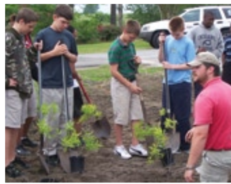
JASON WRIGHT, AN ENGINEER AT N.C. STATE UNIVERSITY, INSTRUCTS STUDENTS OF CHOCOWINITY MIDDLE SCHOOL on building a rain garden.
