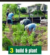
Dig a shallow depression for the outline and base of the rain garden, making sure the bottom depth is at least 1-2 feet above the water table. It is best to plant your rain garden with native plants in the spring or fall when the plants will establish most easily.
