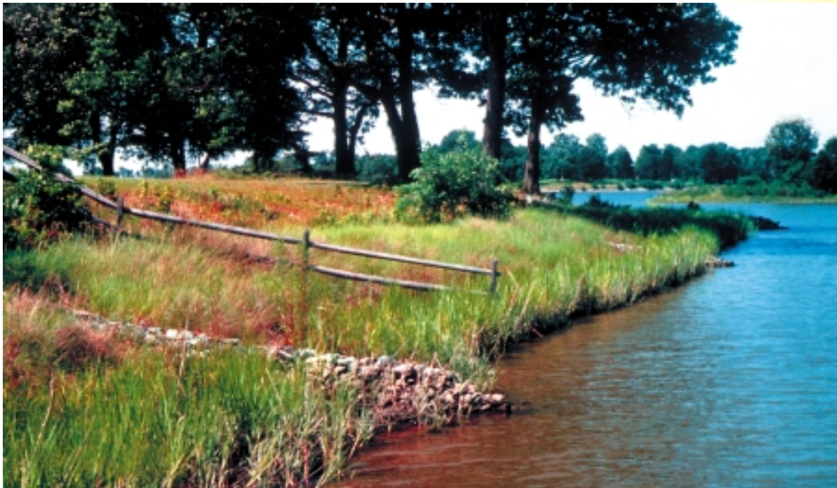
This combination of rip-rap groins and marsh plants create stable areas for successful marsh growth in low energy levels.
