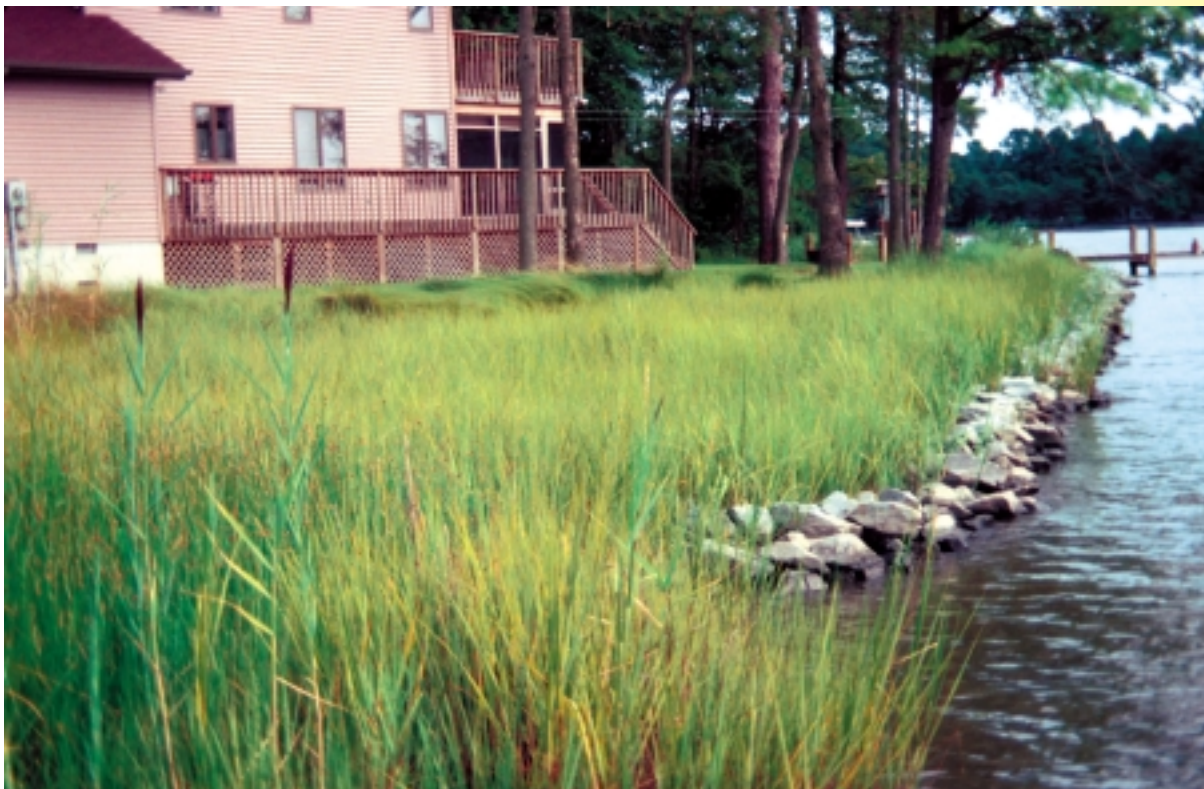
This combination of stone rip-rap and vegetation can be used to provide effective shoreline stabilization.
