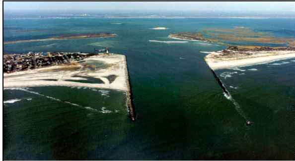
Figure 2. Navigational Jetties (Source: U.S. Army Corps of Engineers, n.d.)
