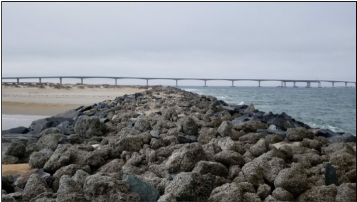
Figure 7. Terminal groin at Pea Island, NC. Photo by Sam Walker.
