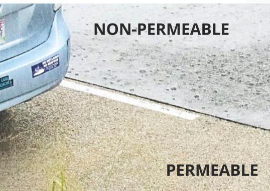
Notice how rainfall soaks into permeable pavement
