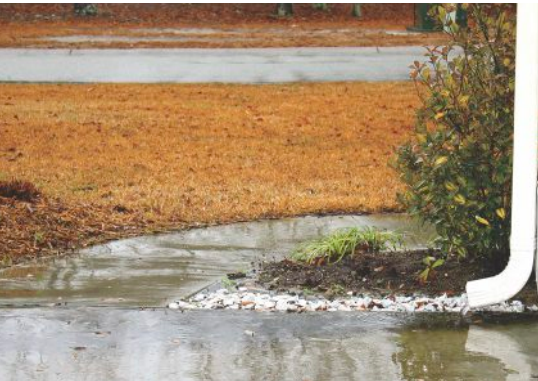
Typical placement of a downspout
