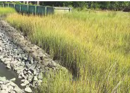
Pine Knoll Shores residential shoreline after restoration
