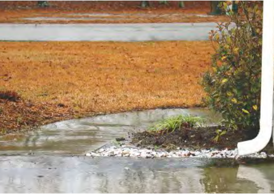
Typical placement of a downspout
