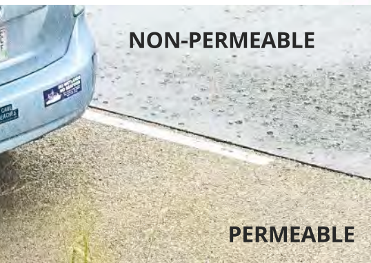
Notice how rainfall soaks into permeable pavement
