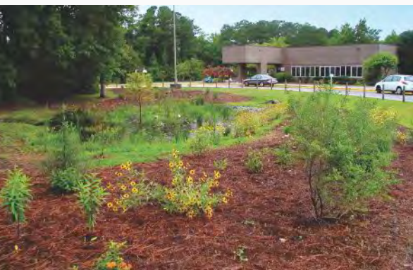
Bradley Creek Elementary School stormwater wetland
