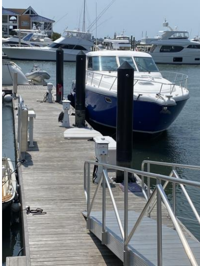
“Telescoping” encapsulated concrete pilings
