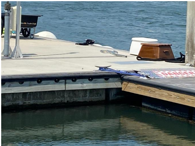
Concrete docking (with concrete floats) and Encapsulated Floating Dock
