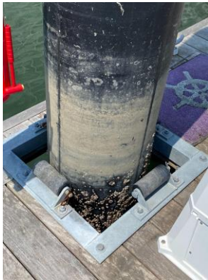
Pile supports/bumpers installed by Bellingham Marine
