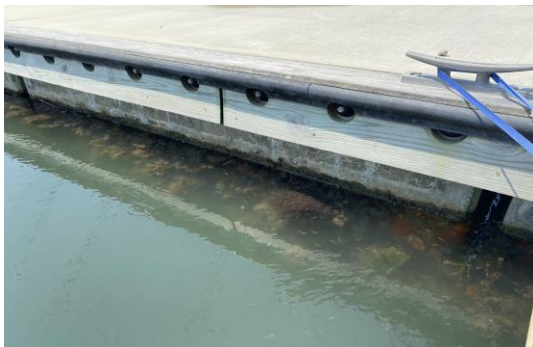
Concrete/timber docking with concrete encapsulated floats
