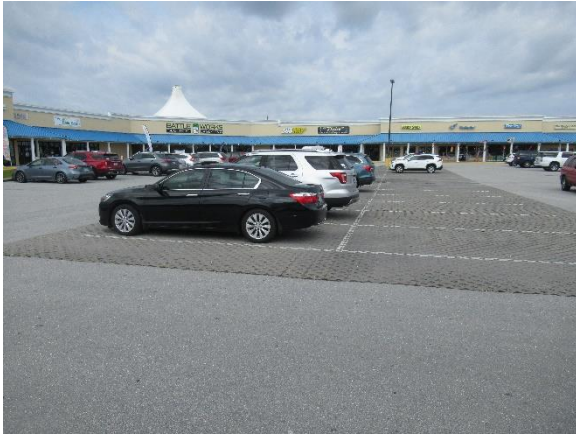
Existing pervious pavement cutouts
