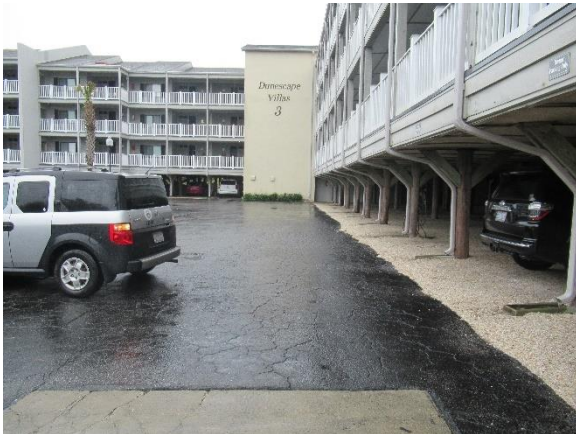
Rooftop downspouts discharging into parking lot
