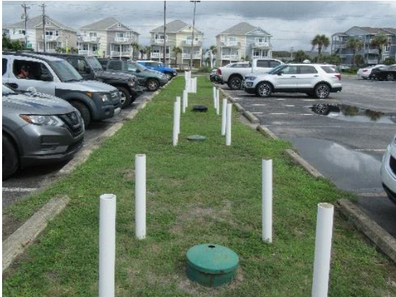
West parking lot at Hilton Double Tree
