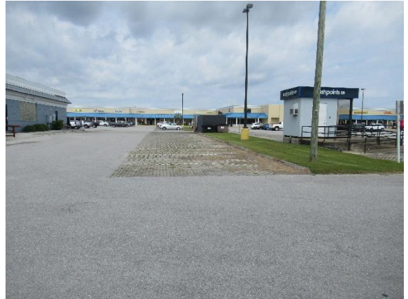
Existing pervious pavement cutouts
