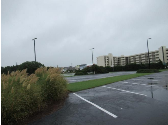
Degraded pavement and stormwater ponding
