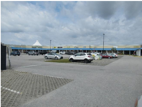
Existing pervious pavement cutouts
