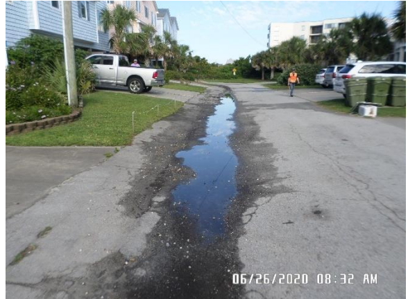
Heavily degraded pavement and stormwater ponding
