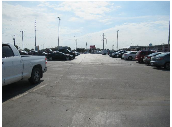
Facing South East showing large parking lot that drains directly into Bogue Sound
