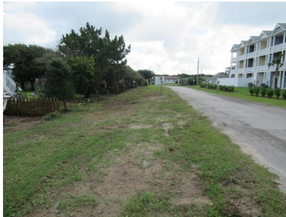
Roadside grass experiencing erosion from stormwater
