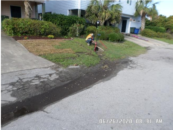
Heavily degraded pavement not draining into stormwater infrastructure
