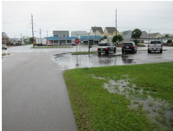
Excessive stormwater ponding in parking lot
