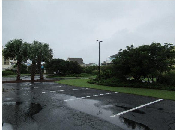
Degraded pavement and stormwater ponding
