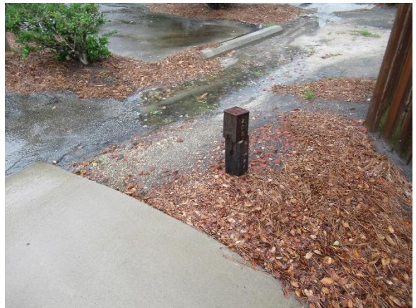
Sediment buildup and erosion from stormwater
