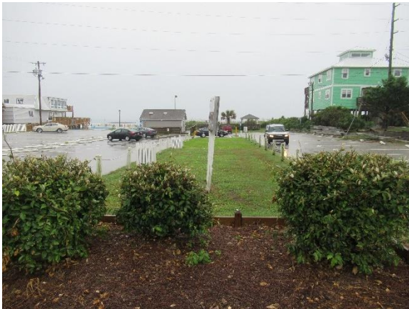
Parking lot experiencing stormwater ponding
