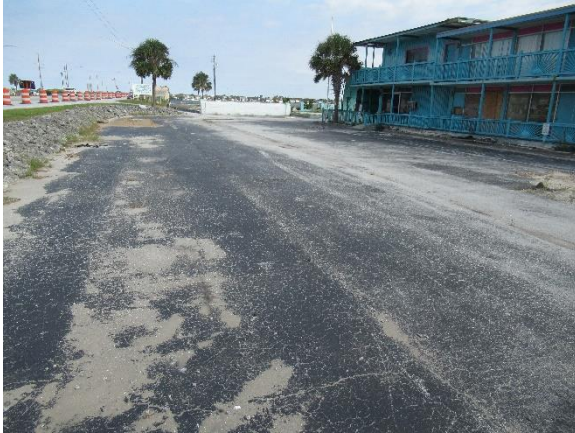
Degraded parking lot in front of building
