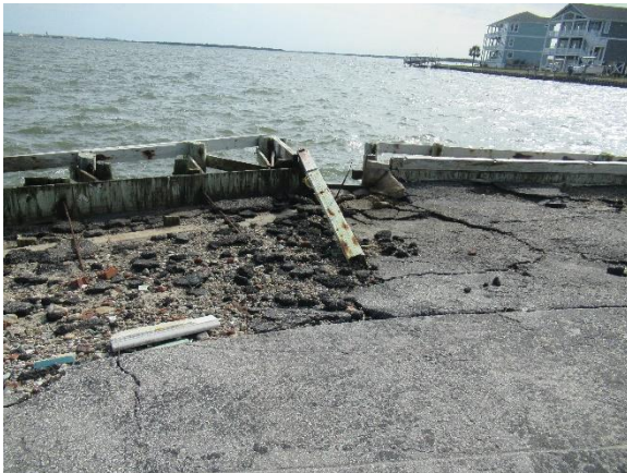
Direct outlet to Bogue Sound on North West corner of parking lot
