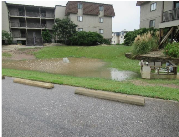
Stormwater erosion and ponding
