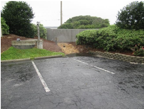
Degraded pavement and stormwater pipe
