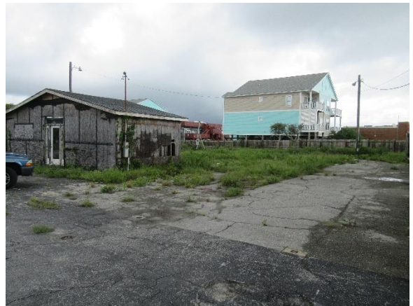
Degraded parking lot behind Kitty Hawk Kites
