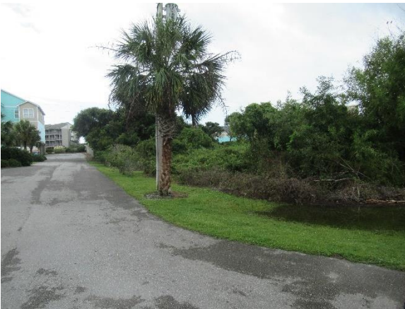
Ponding on the corner of undeveloped lot
