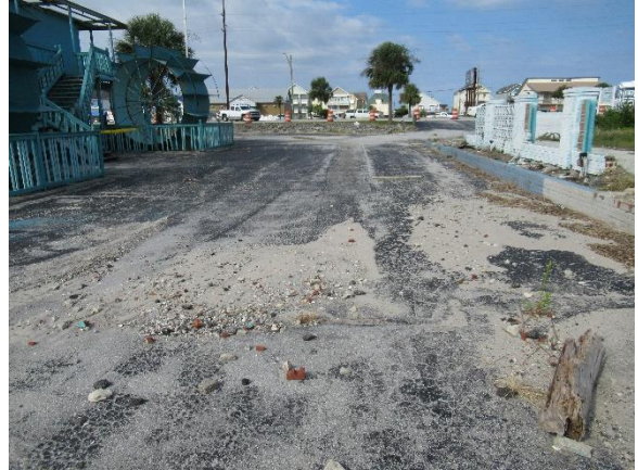
Sediment accumulation at low point on North side of building
