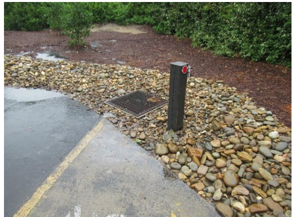
Existing drop inlet
