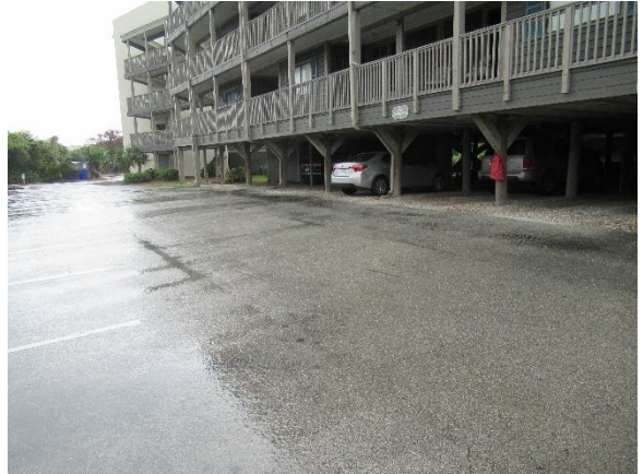
Roof downspouts flowing into parking lot
