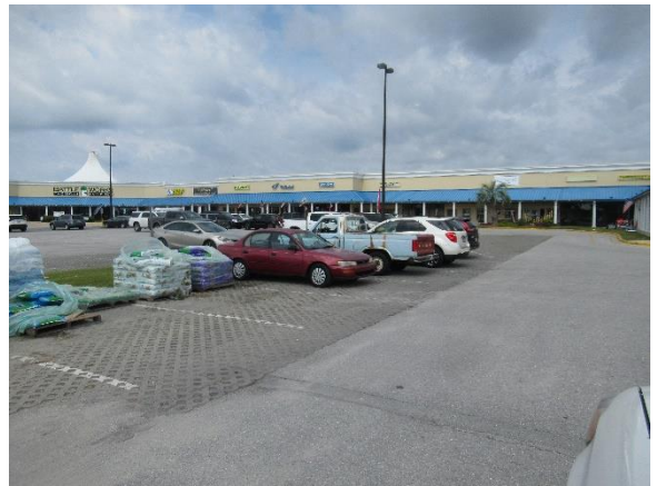
Existing pervious pavement cutouts
