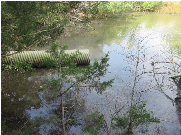
Large CMP discharging into Hoop Pole Creek
