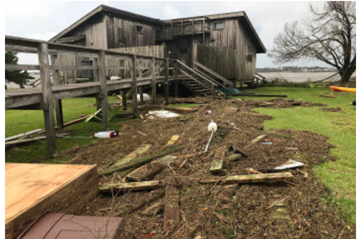
Near Harkers Island Bridge shortly after Hurricane Florence hit in 2018. Photo: Lillie Chadwick Miller
