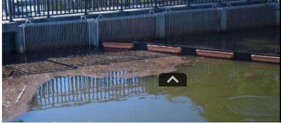
Carp barriers cut in half are easier to lift to flush debris
