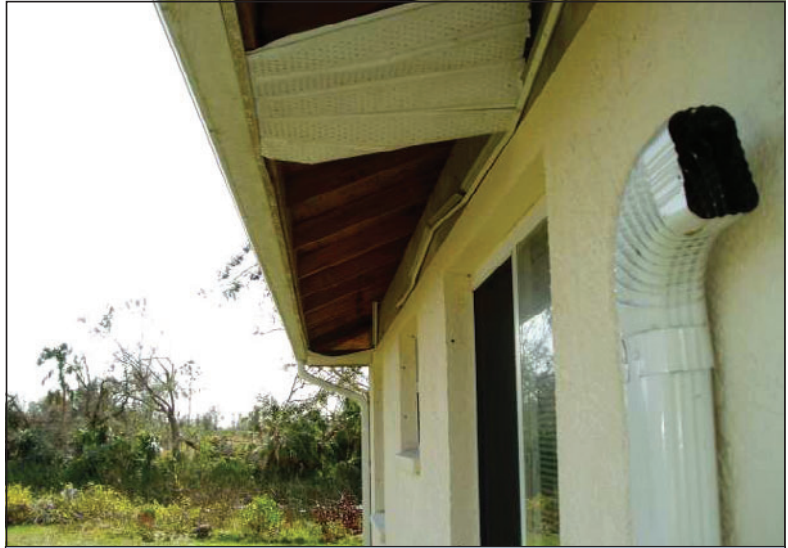
Figure 1. Missing soffit material.
