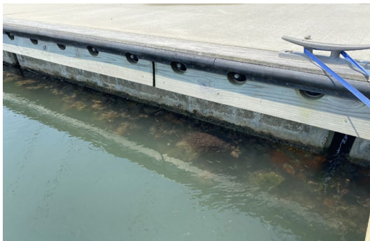
Concrete/timber docking with concrete encapsulated floats
