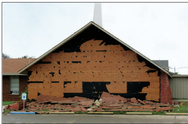
Figure 1. Failed brick veneer over plywood. Many of the ties are still attached to the substrate, but several of the tie fasteners pulled out of the substrate and the ties are embedded in the collapsed veneer. Estimated wind speed: 107 miles per hour (peak gust, Exposure C, at 33 feet).
