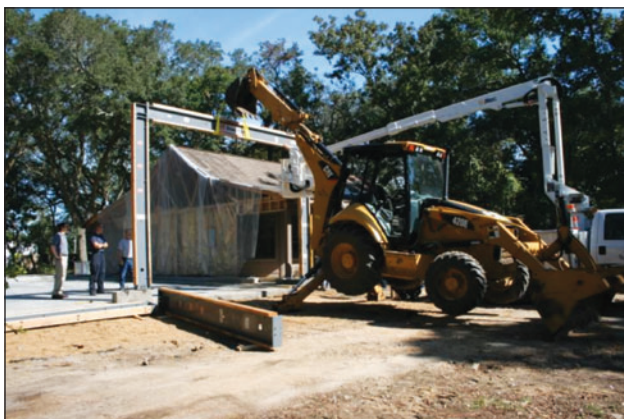
Figure 4. Installation of a prefabricated ordinary moment frame.
