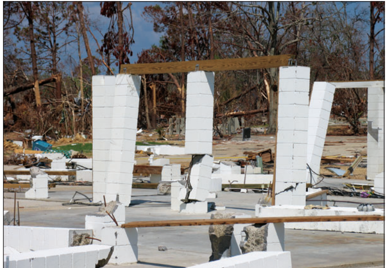
Figure 2. Pier breakage (Long Beach, Mississippi)
