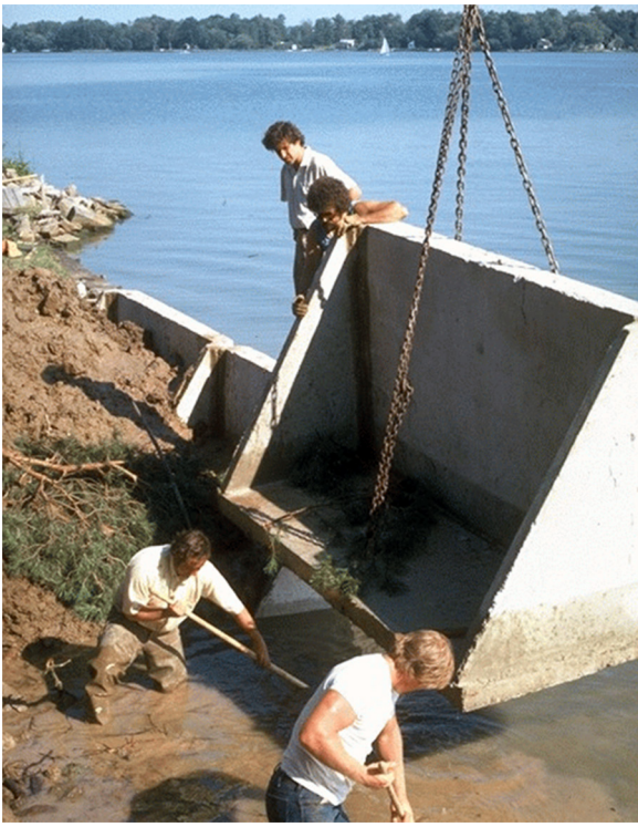
Figure 2. A precast concrete bulkhead is assembled on the shore of a Lake Ontario embayment.
