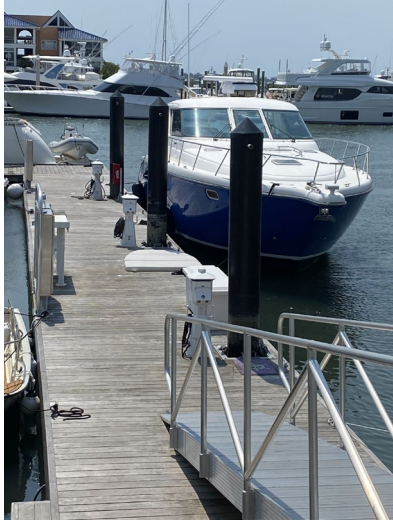
“Telescoping” encapsulated concrete pilings
