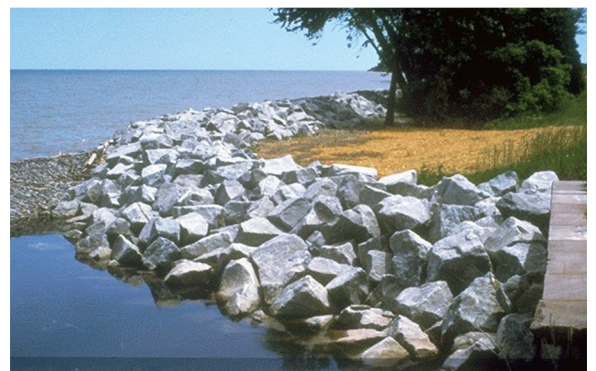
Figure 4. A dolomite revetment construction to protect the Lake Ontario State Parkway from the ravages of stormwaves.
