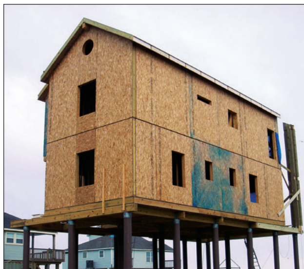
Figure 2. Construction of a Structural Insulated Panel house.
