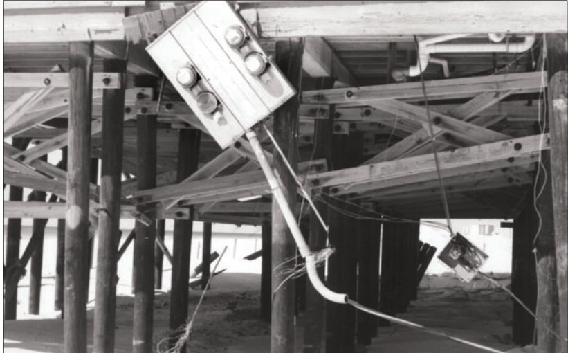
Electrical lines and box dislocated by hurricane forces.
