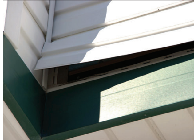
Figure 4. Utility trim was substituted for the starter strip and the bottom lock was cut off the siding. Siding was able to pull loose under wind pressure.
