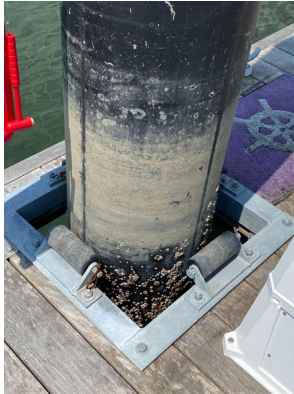
Pile supports/bumpers installed by Bellingham Marine
