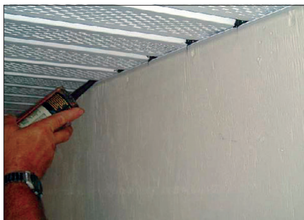
Figure 4. Applying dabs of sealant.
