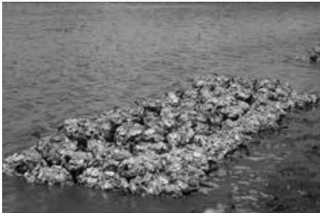
**Oyster shell bags** are plastic mesh bags filled with fossilized and/or recycled oyster shell. Because loose shell can be more easily moved by waves before growth of new oysters can occur, loose shell is packed in aquaculture grade mesh bags before being used in oyster reef creation.
