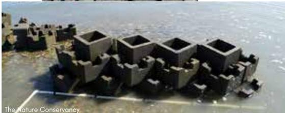
**The Oyster Castle®** is an easily deployed, specialized manufactured concrete unit using an environmentally friendly, certified blend of material conducive to fostering oyster settlement, attachment, and growth.
