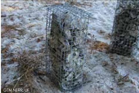
**Oyster gabions** are wire cages filled with recycled oyster shell. Gabions are great for shallow tidal creeks, bays, brackish rivers, and marsh lands. The gabions provide spat with a safe and healthy place to grow, while helping protect against erosion and scour.
