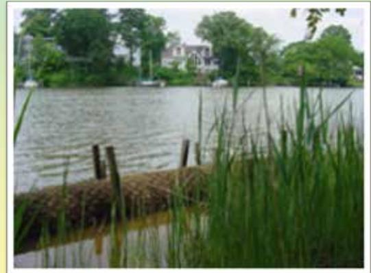
In areas with minimal wave energy; plantings with temporary protection, in the form of fiber-logs can provide temporary protection while the plants are growing/maturing; these work best in freshwater applications and can provide energy dissipation for up to 18 months, which should allow the plants the time necessary to coalesce. These applications do need initial monitoring and likely some maintenance to ensure that the plants are growing and expanding as anticipated!
