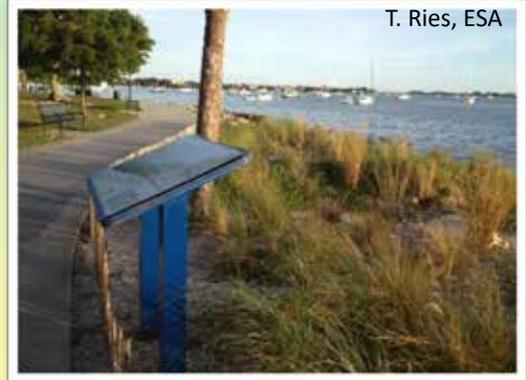
Planted Shoreline - the easiest and least cost expensive option is just regrading the eroded slope and planting with native vegetation, which worked at this site in Sarasota Bay; however, if there was an eroded bank, the cause of the erosion **must** be addressed (e.g. minimum wake zone enacted or wave energy protection installed) before just installing plants along the shoreline.
