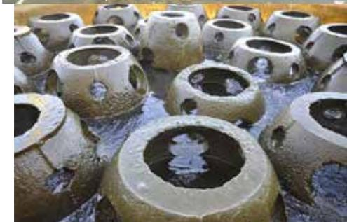
**Oyster reef balls** can be used to decrease wave energy while enhancing fish and oyster habitat. These structures provide a surface on which oysters colonize and form small living reefs. These structures also dissipate waves, decreasing coastal erosion and providing an area in which newly planted vegetation can grow.
