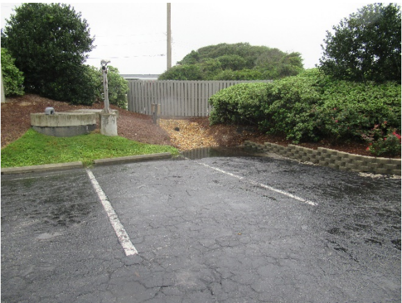
Degraded pavement and stormwater pipe
