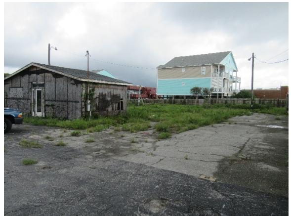
Degraded parking lot behind Kitty Hawk Kites
