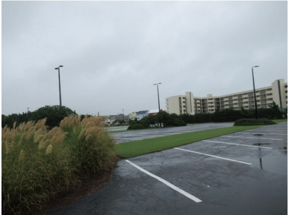
Degraded pavement and stormwater ponding
