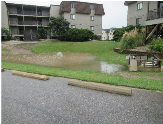
Stormwater erosion and ponding
