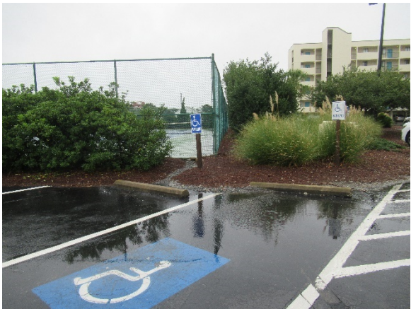
Stormwater runoff from tennis court flowing across mulch and into parking lot
