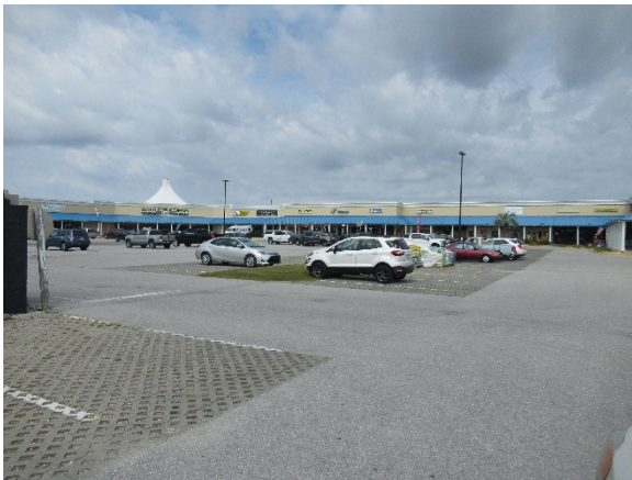
Existing pervious pavement cutouts
