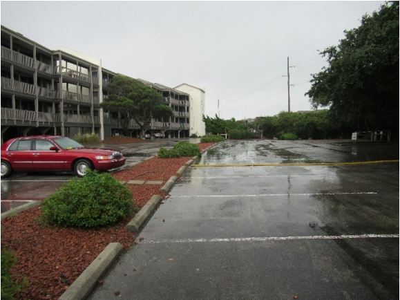
Stormwater ponding
