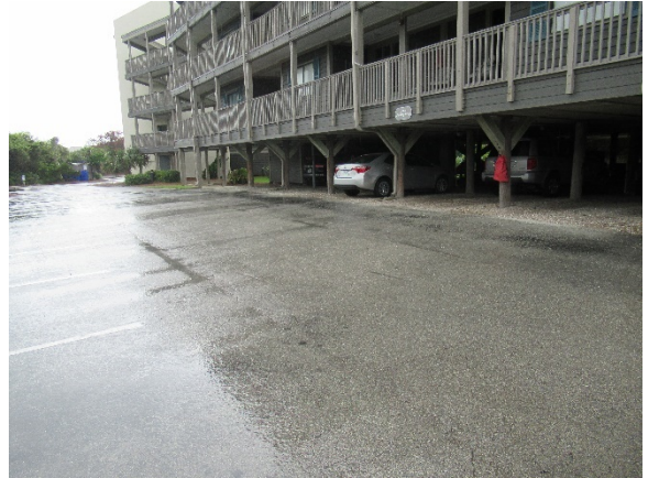
Roof downspouts flowing into parking lot
