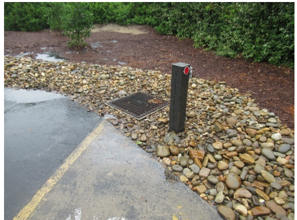
Existing drop inlet
