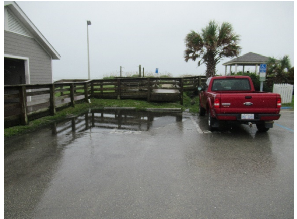
Stormwater runoff from parking lot to the beach
