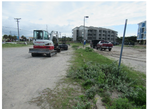
Unpaved lot West of Hilton Double Tree
