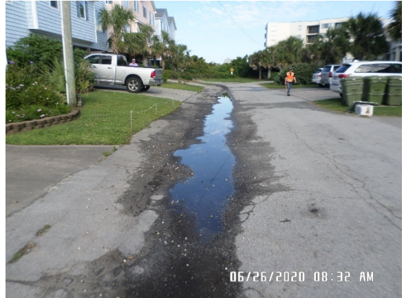
Heavily degraded pavement and stormwater ponding
