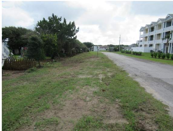
Roadside grass experiencing erosion from stormwater
