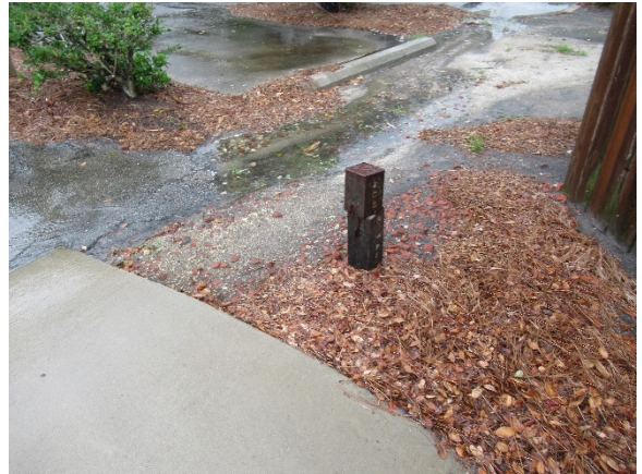
Sediment buildup and erosion from stormwater
