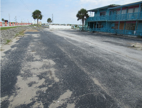
Degraded parking lot in front of building
