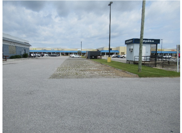
Existing pervious pavement cutouts
