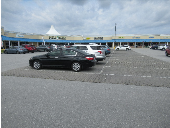
Existing pervious pavement cutouts
