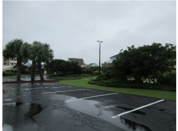
Degraded pavement and stormwater ponding
