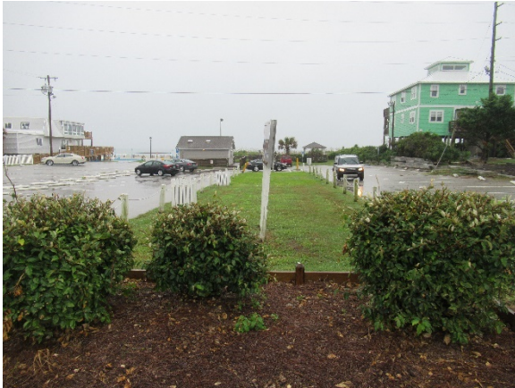
Parking lot experiencing stormwater ponding
