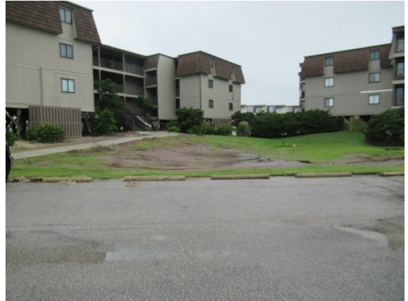
Stormwater erosion
