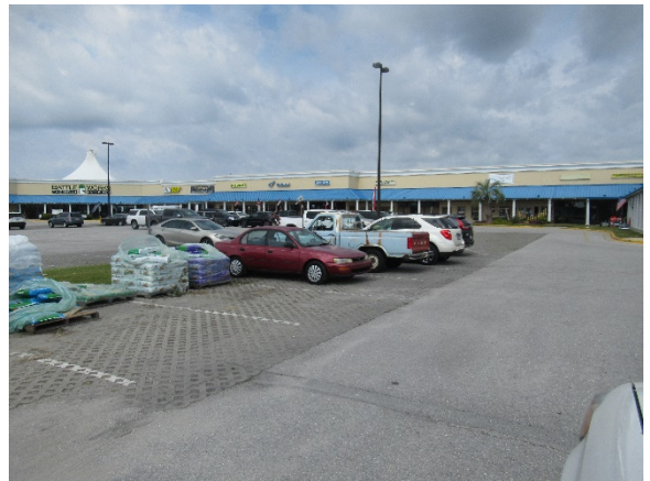
Existing pervious pavement cutouts
