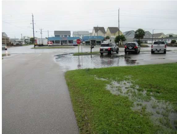
Excessive stormwater ponding in parking lot
