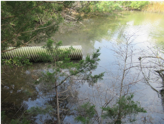
Large CMP discharging into Hoop Pole Creek
