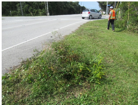
Side of road draining into Hoop Pole Creek
