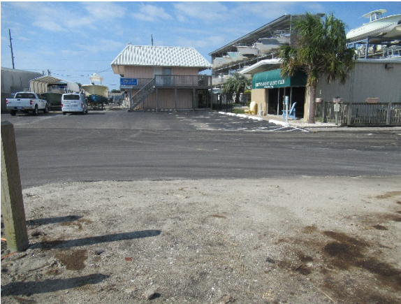
Facing West from drop inlet
