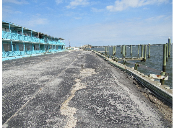
Degraded pavement and sediment accumulation on West side of building
