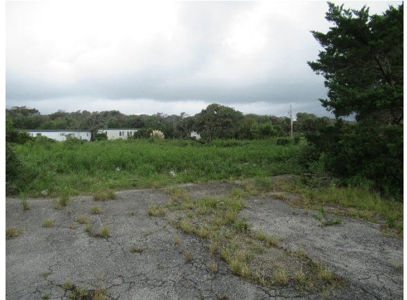
Parking lot draining to undeveloped lot
