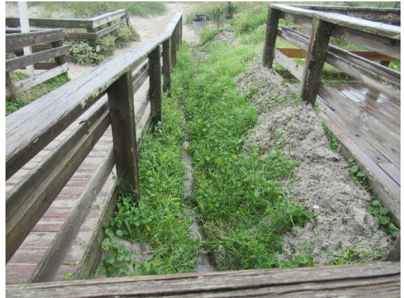
Channelized flow from parking lot to the beach
