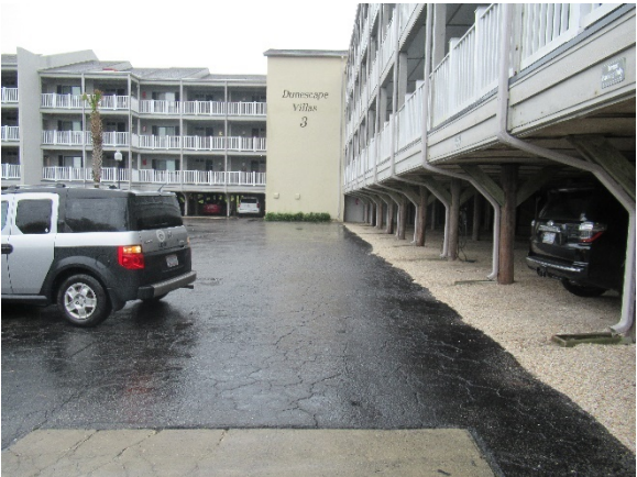
Roof downspouts discharging into parking lot
