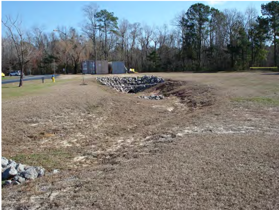
Photo 2. Eroding ditch with closely cut grass
