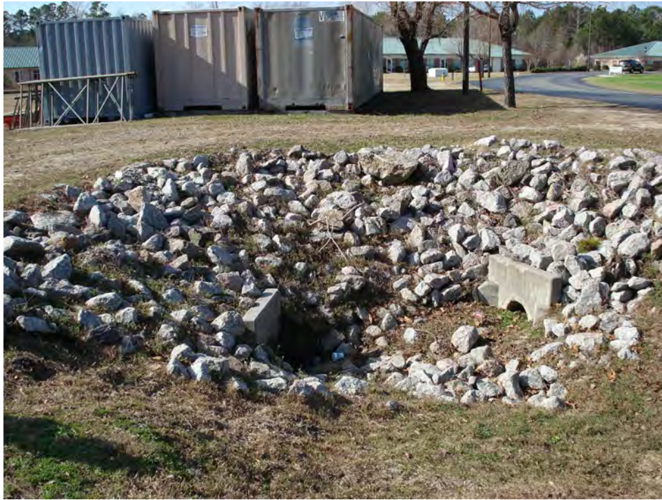
Photo 5. Culverts filling in the sediment
