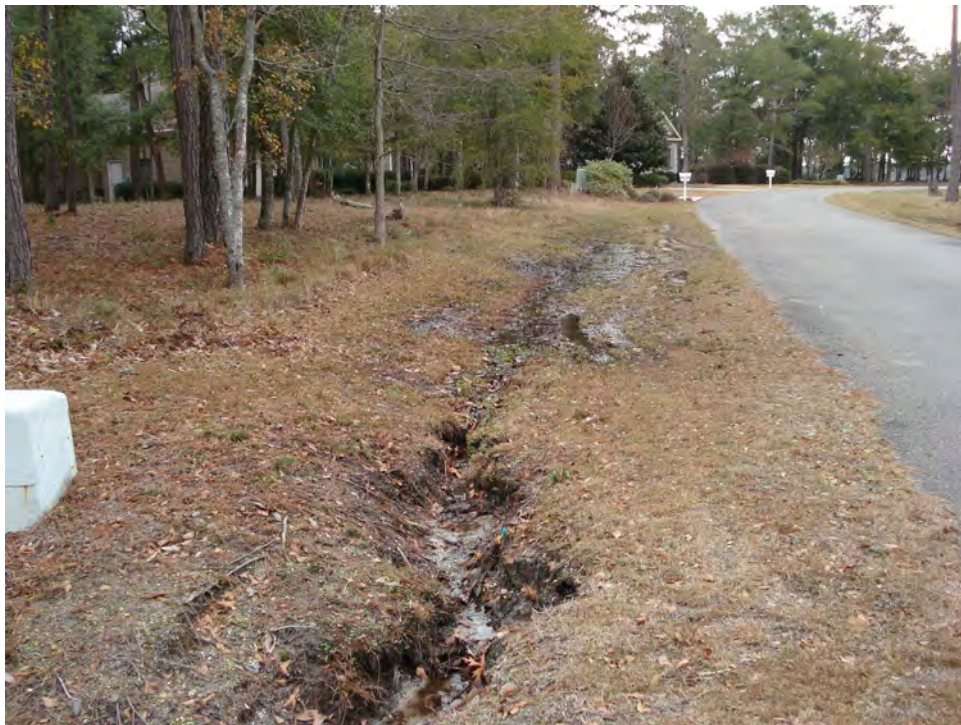
Photo 2. Erosion along roadside due to stormwater flow
