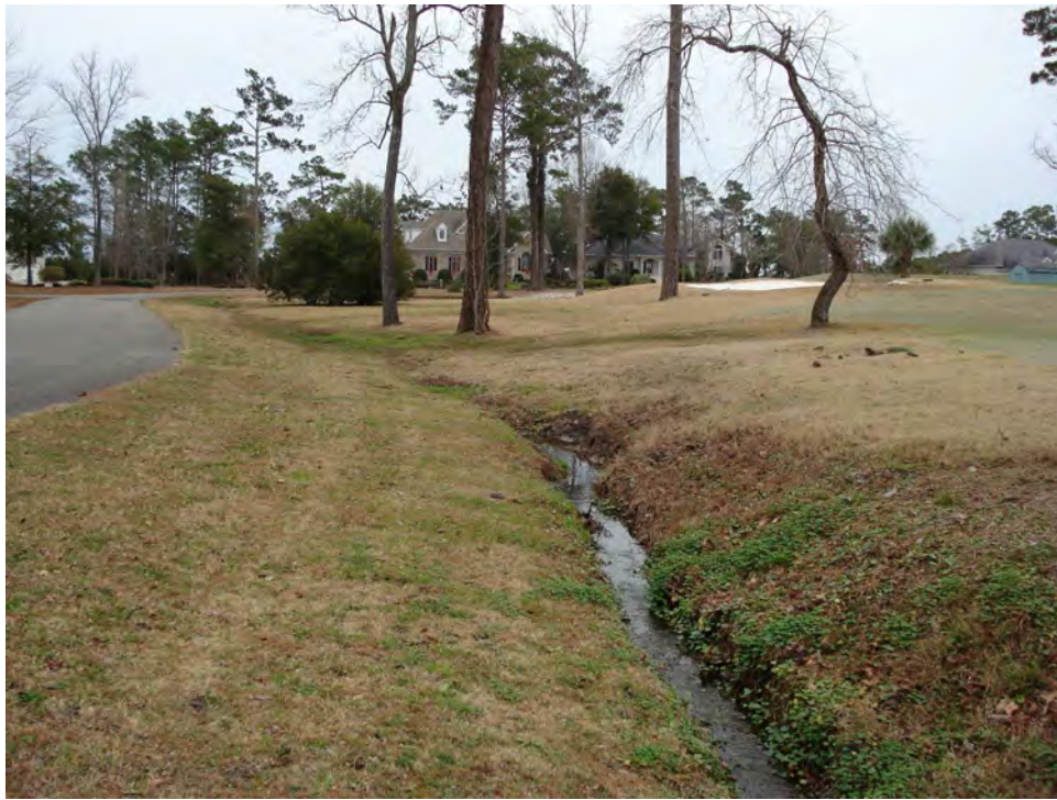
Photo 3. Ditch forming along roadside, discharges into LFR inlet
