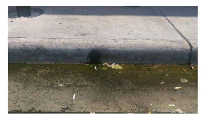
Figure D-7. High volume drainage into Front Street near Clawson's, from the building's green roof.
