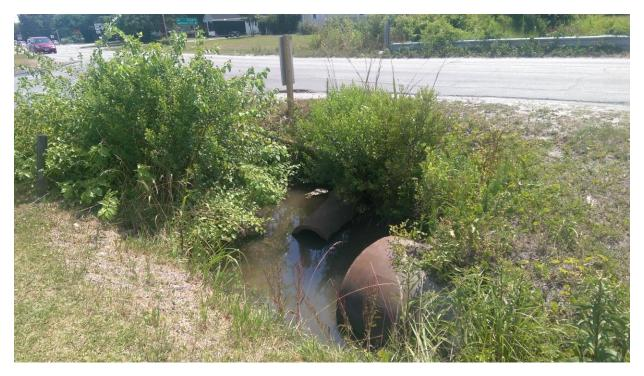
*Figure D-7: Example of areas that may have problematic drainage along Route 101.*
