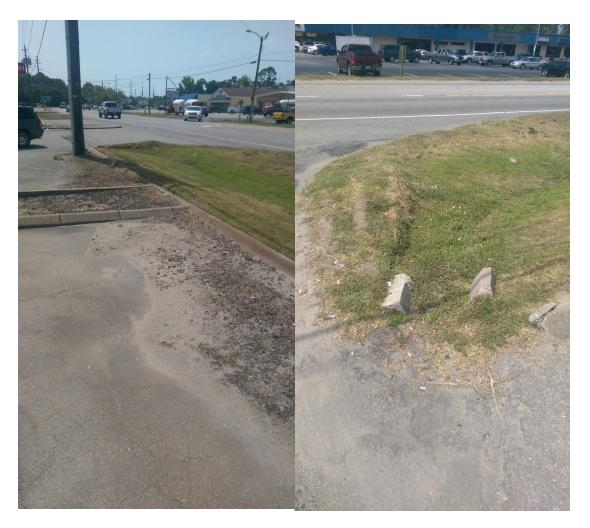
Figure D-5: Examples of areas that could benefit from curb cuts and grading along Highway 70.
