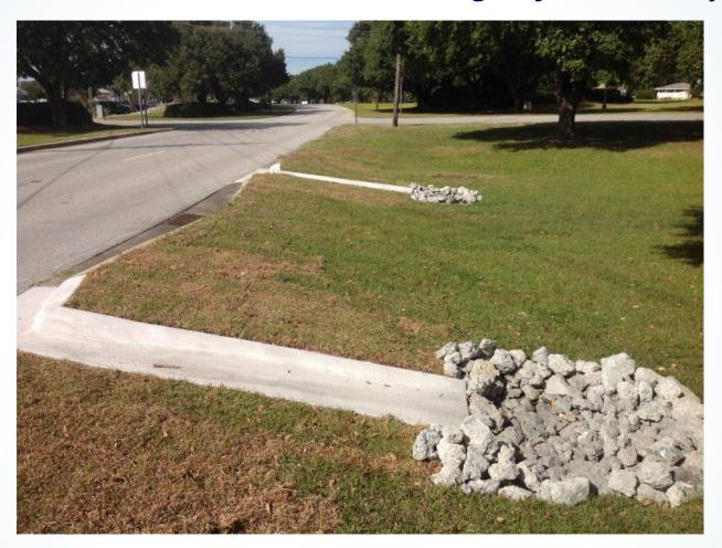
With a slight change to the landscaping and the addition of two curb cuts and a raised drain, runoff is directed into the grassy median where it soaks slowly into the ground reducing flooding and discharge to surface waters.
