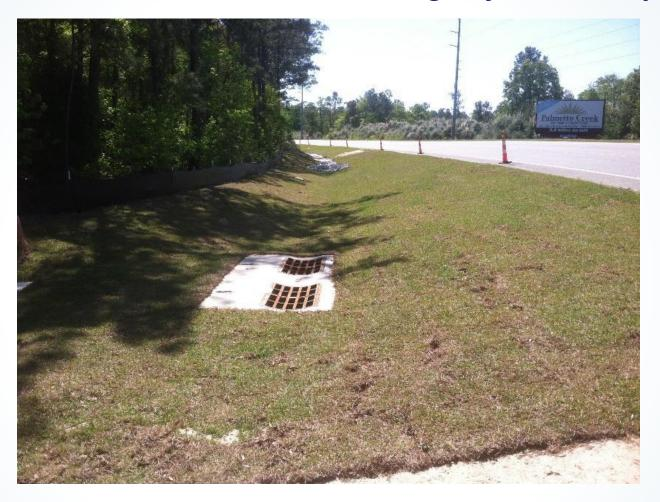
The bioswale (background) infiltrates runoff from Hwy 211 and reduces pollutants entering the Lockwood Folly River while the bioswale outlet (foreground) structure captures overflow during heavy rain events.
