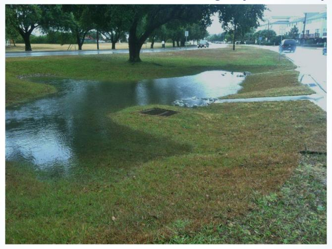
Stormwater is directed from the street to the grassed median. An overflow is raised to give the rain a chance to soak in.
