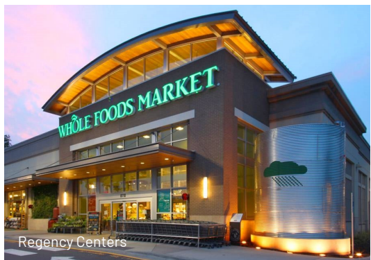
An underground detention chamber, bioswales, and cistern are three types of nature based strategies used at the Market of Colonnade site.
