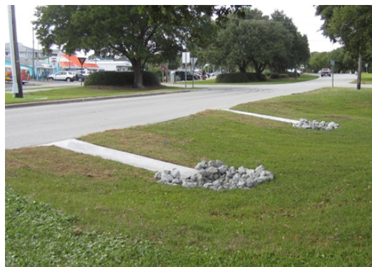
Water is directed to the curb cuts and feeds into vegetated areas where it can infiltrate the soil.
