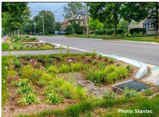
Roadside stormwater infiltration techniques collect rain to reduce runoff.
