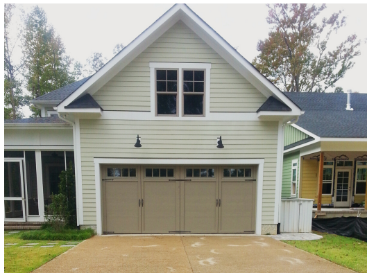
Permeable pavement infiltrates rain to reduce runoff in New Hanover County.
