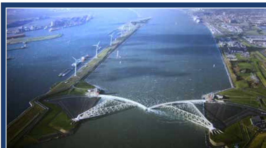
The Maeslantkering is a storm surge barrier in South Holland, Netherlands and one of the largest moving structures on Earth. It is automatically triggered by a supercomputer to close when Rotterdam is threatened by floods. Photo: maaslant kering (5) by bertknot via Flickr
