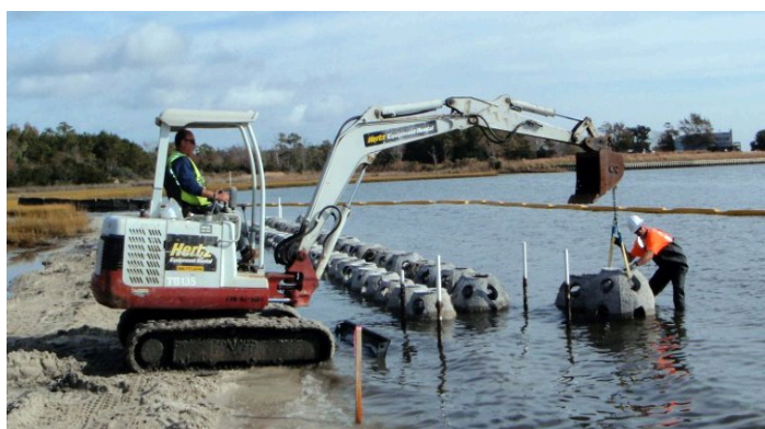
Figure 8-1. A contractor places oyster domes into the sound as part of a living shoreline installation.
