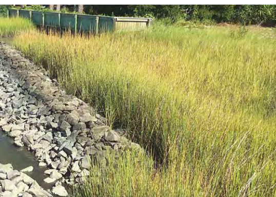
Pine Knoll Shores residential shoreline after restoration
