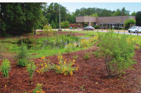
Bradley Creek Elementary School stormwater wetland
