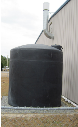
WESTERN CARTERET FIRE AND EMS CISTERN
