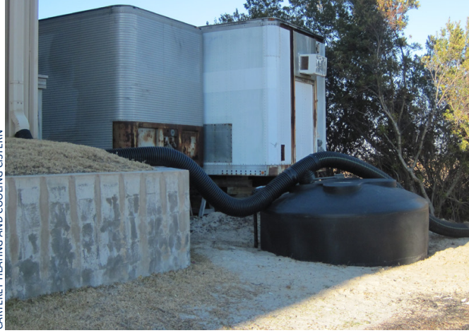
CARTERET HEATING AND COOLING CISTERN
