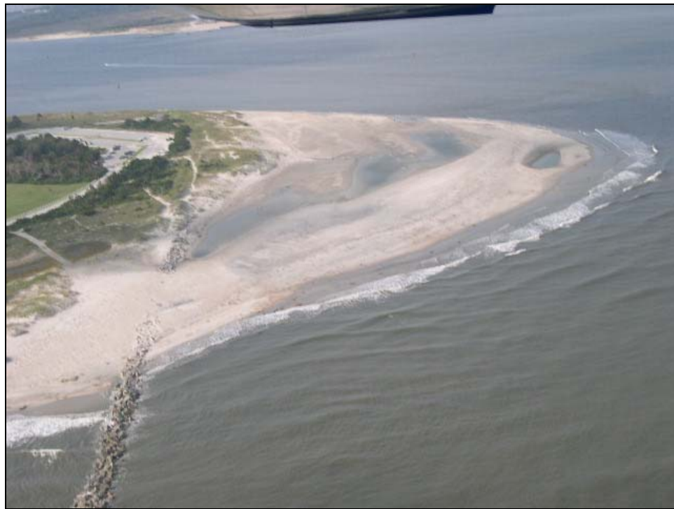
Figure 12. Sand spit growth showing the inability of the terminal groin to trap sediment.
