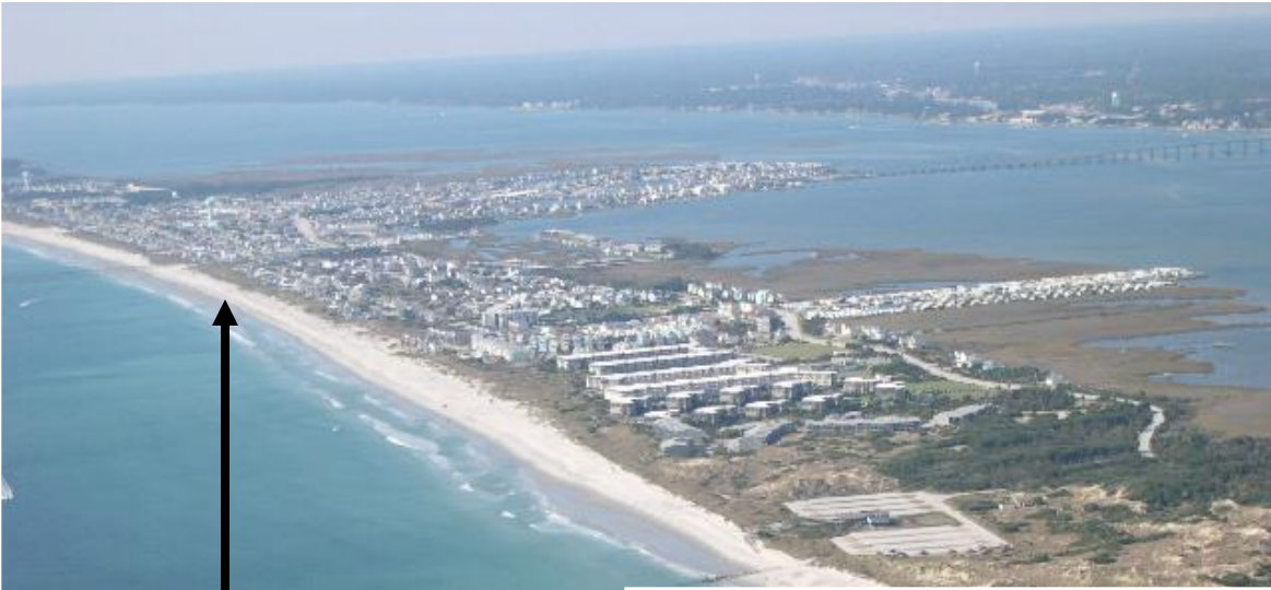
DOWNSTREAM SHORELINE RECESSION AT ATLANTIC BEACH
