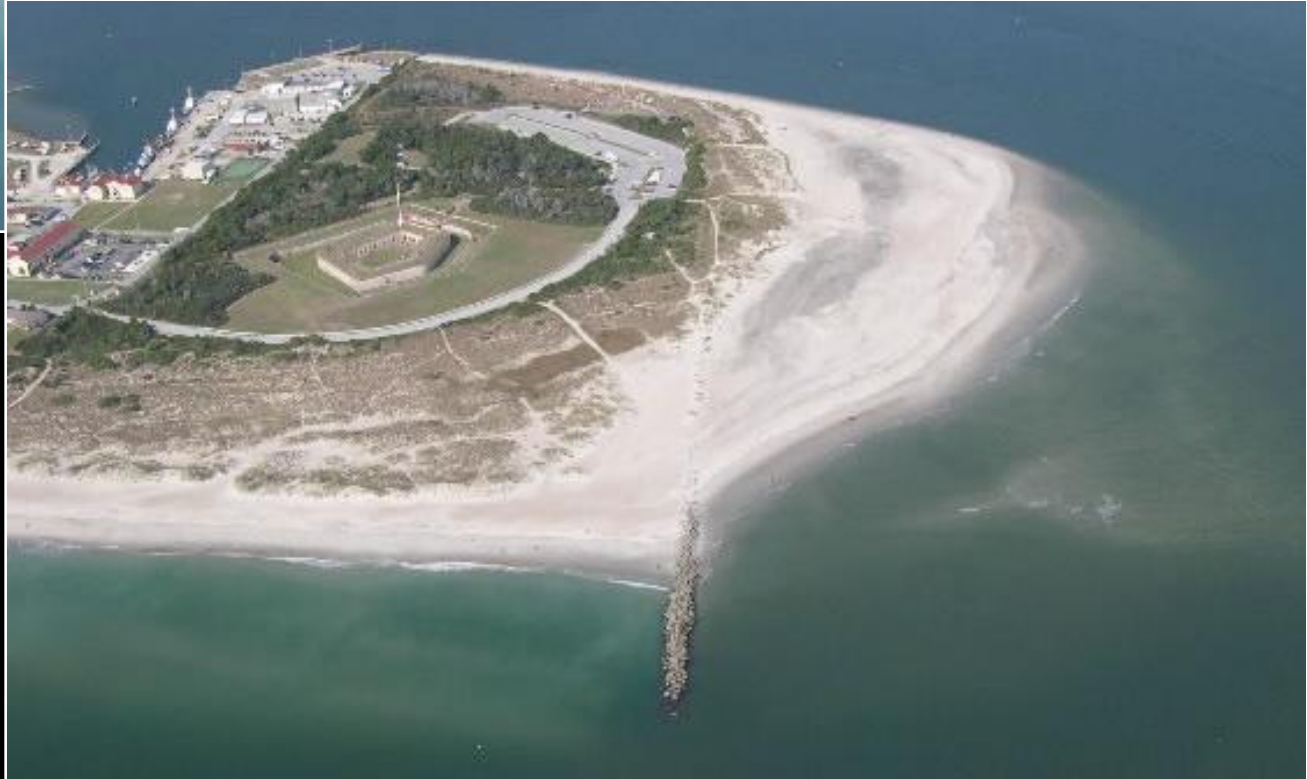
BEAUFORT INLET TERMINAL GROIN AT FORT MACON
