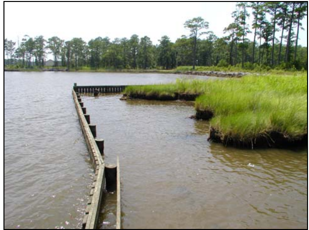
Figure 5-6: View of a rubble mound (rock) sill (left) and a timber sheet pile sill (right).
