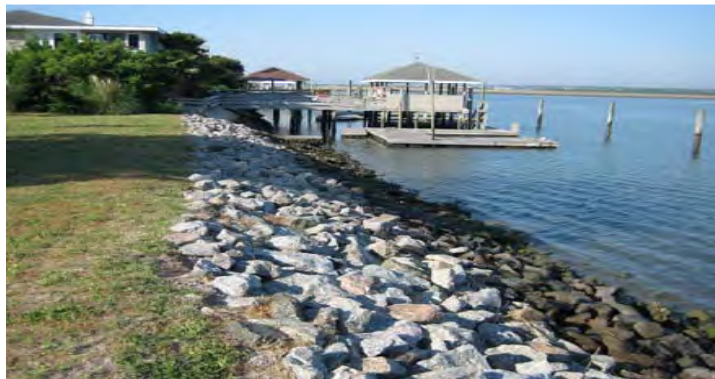
Revetment (Photo: N.C. Division of Coastal Management)
