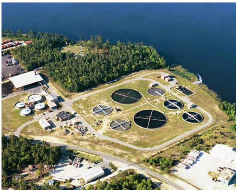
McKean-Maffit (Southside) Wastewater Treatment Plant in Wilmington 329
