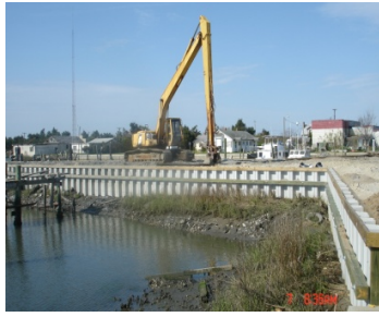
Bulkhead under construction
