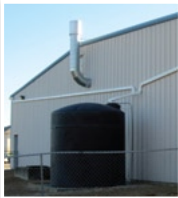
The cistern at Western Carteret Fire Department
