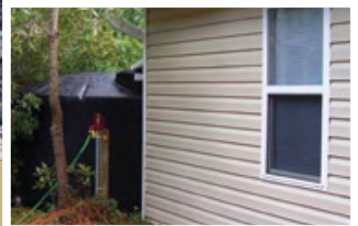
above: Oyster shells that the federation puts in bags to create reefs are at a premium. right: The federation installed this cistern behind our Learning Center to capture rooftop runoff.
