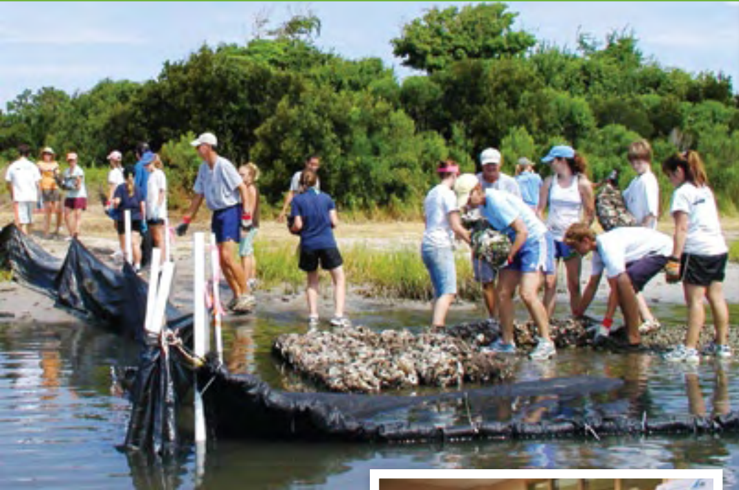
left and above: Volunteers form a line to build an oyster sill at Morris Landing in Onslow County and then plant marsh grasses to stabilize the shoreline.
