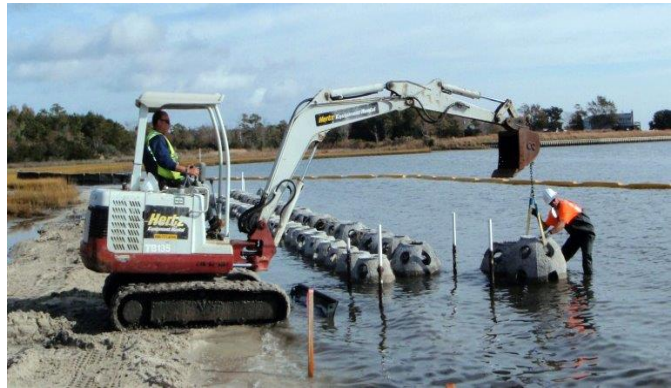
Figure 8-1. A contractor places oyster domes into the sound as part of a living shoreline installation for a 2011 coastal watershed management plan.
