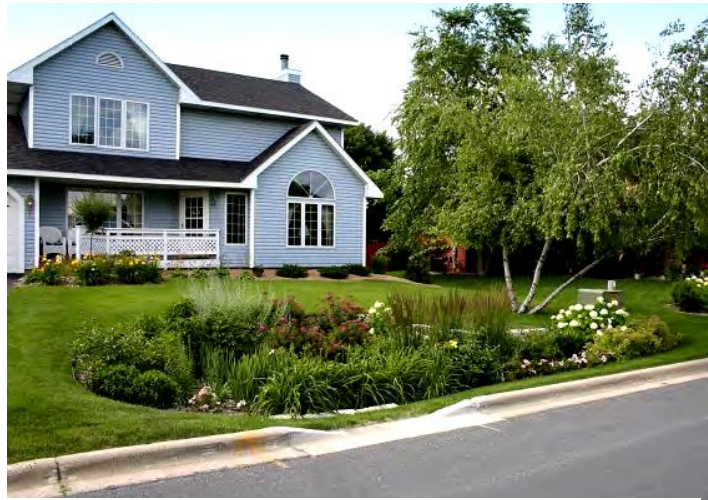
Figure 7-3. A house with a rain garden utilizing native landscaping. Notice the curb cut that allows street runoff to reach the rain garden.
