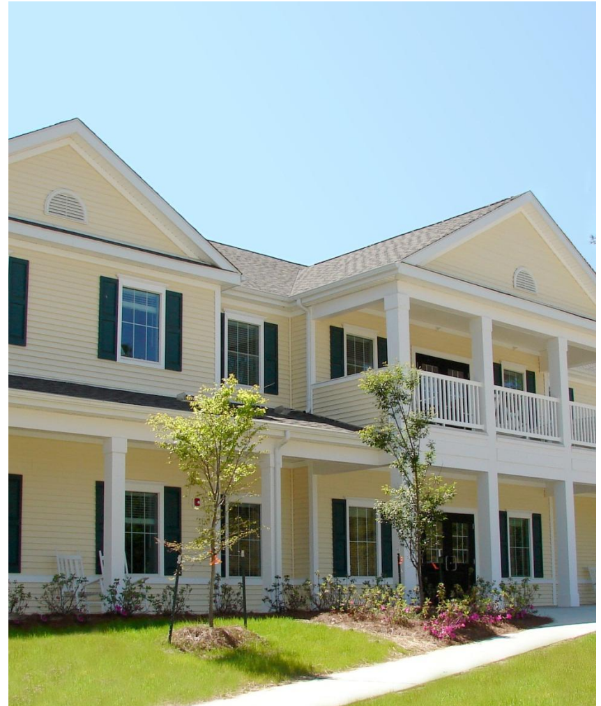
Atlantic Marine Corps Communities, Tarawa Terrace Community Center
