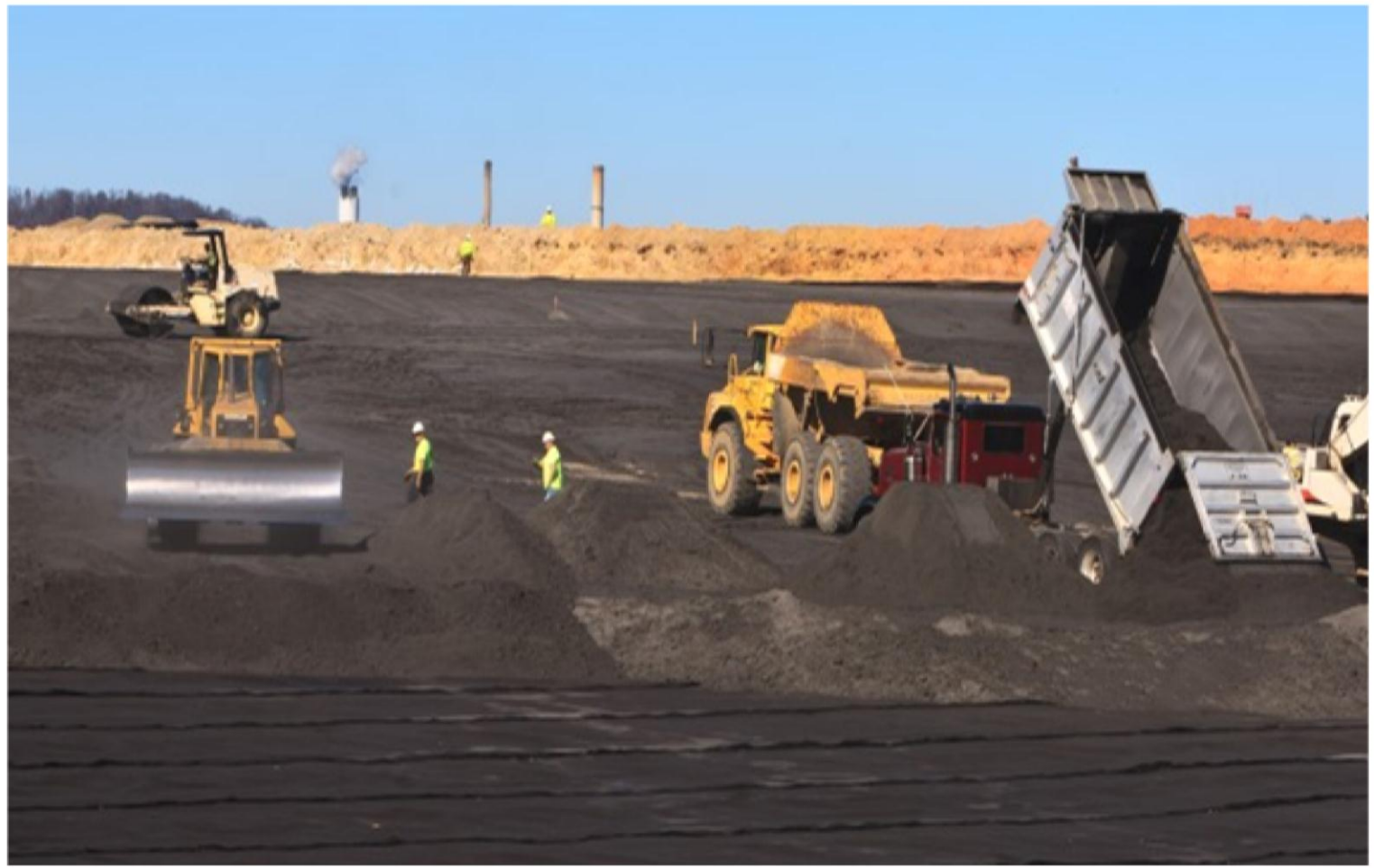
Ash placement over liner system
