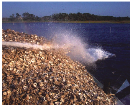
Spreading of oyster shells for new reef base.
